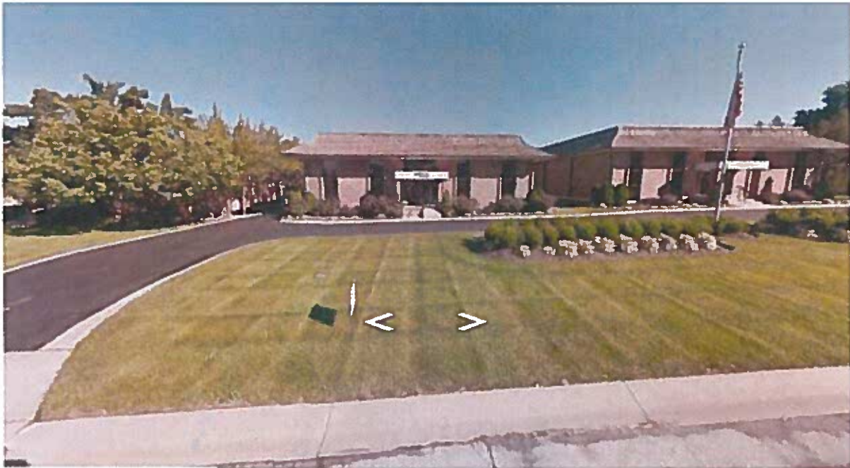
Street view of site frontage area
