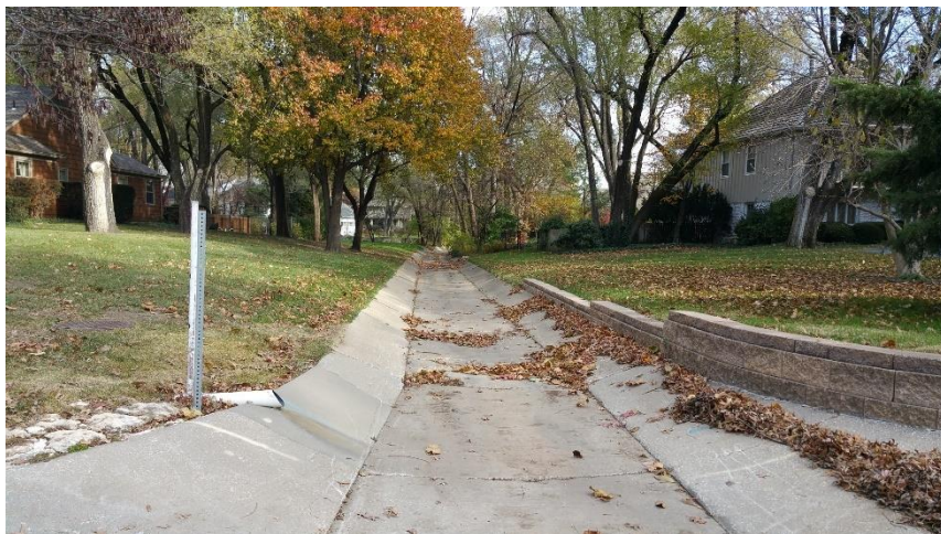
Figure 7 Looking Downstream from Fontana Street
