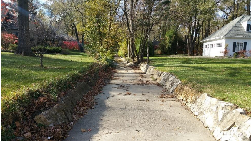
Figure 5 Looking Upstream for Delmar Lane
