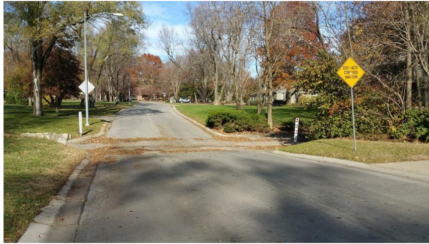
Figure 8 Delmar Low-Water Crossing
