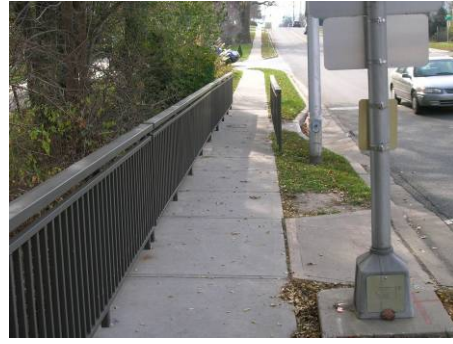
Example of a pedestrian railing
