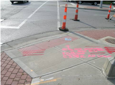
Example of an ADA compliant sidewalk ramp
