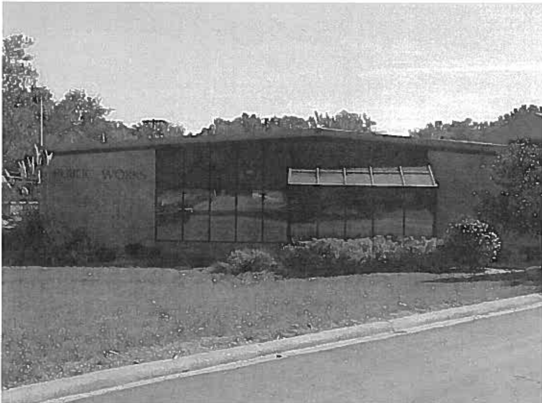
Public Works Office, 3535 Somerset Drive
