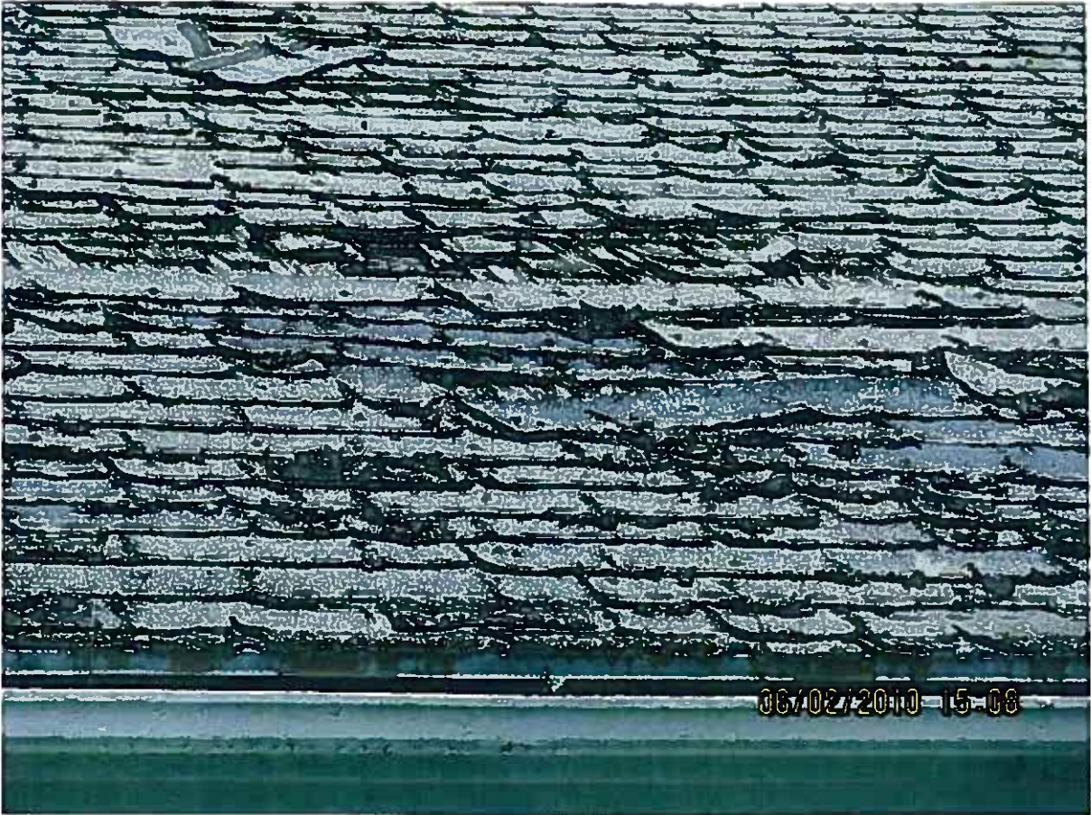
Various roof areas.
