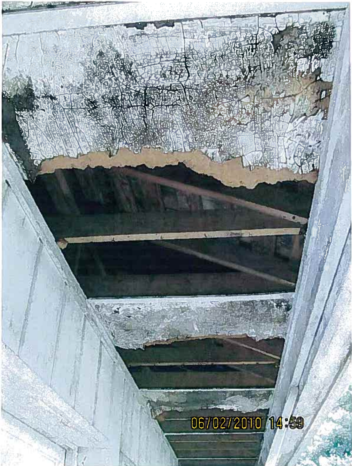
Soffit area in front of garage.
