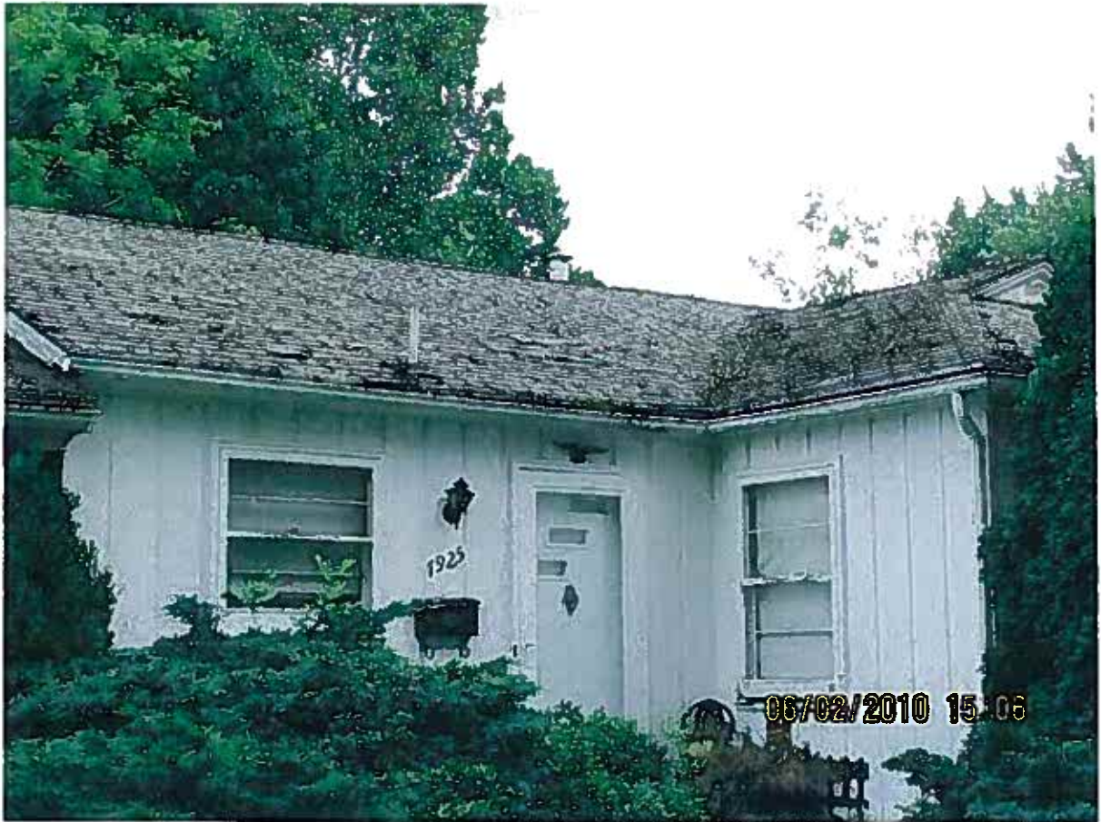
Various roof areas.
