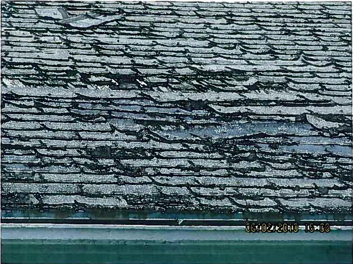
Various roof areas.
