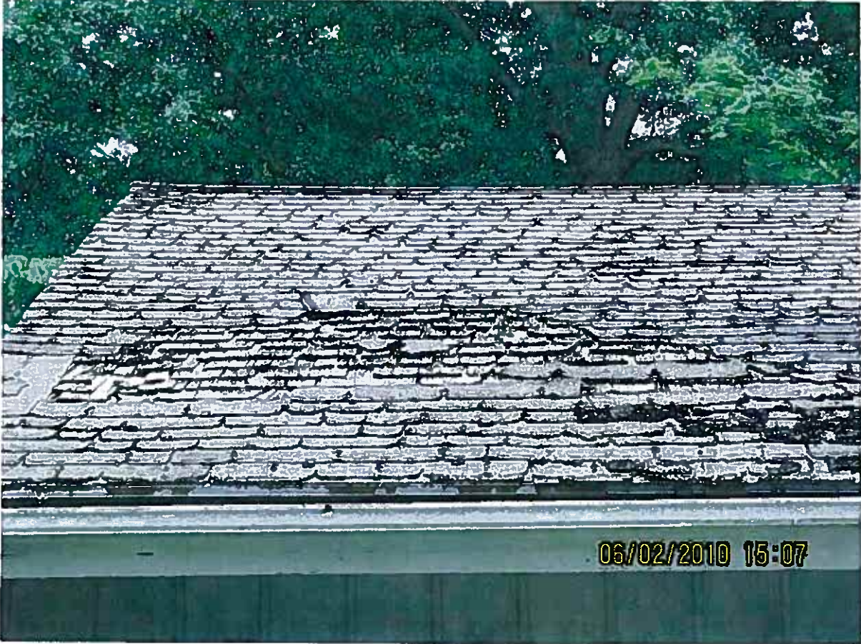
Various roof areas.
