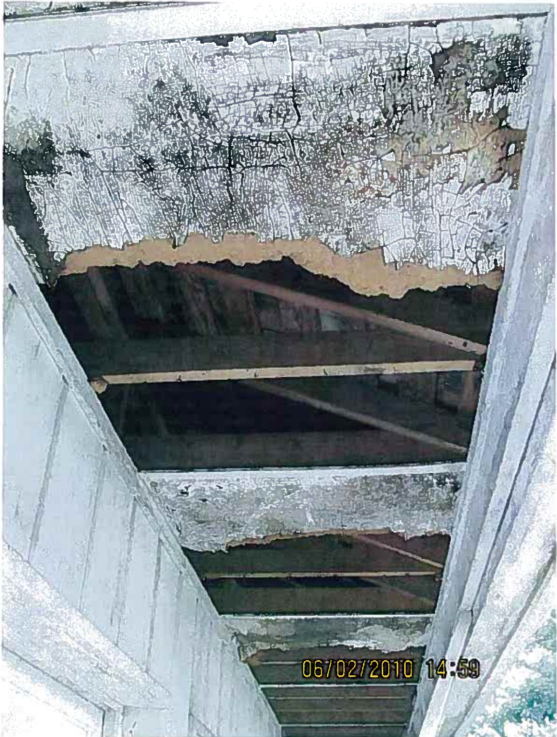
Soffit area in front of garage.
