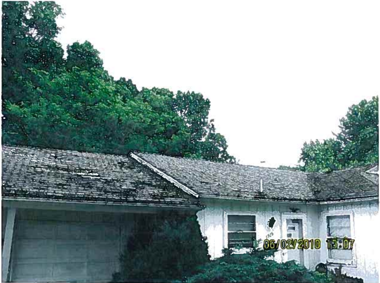
Various roof areas.
