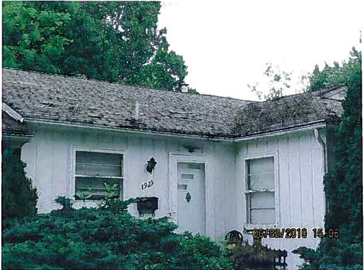
Various roof areas.
