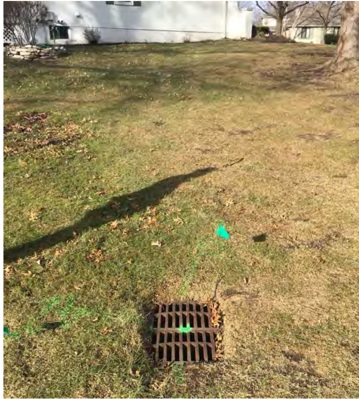
Figure 3 – Typical Backyard Grate Inlet
