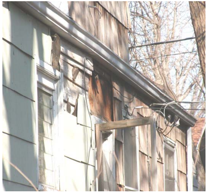
Missing shingles
