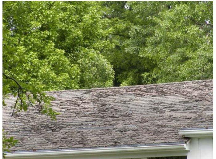
Deteriorated Roof
