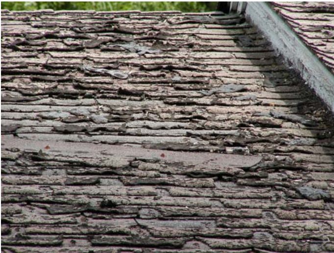
Deteriorated Roof
