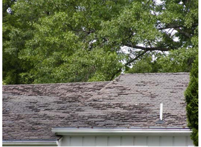
Deteriorated Roof
