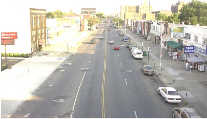
4 Through Lanes, No Bike Accommodation
