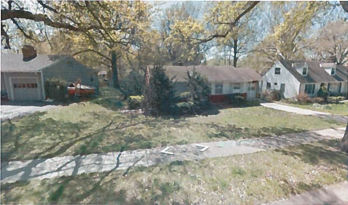
Existing street view 2907 W. 71 st Terrace
