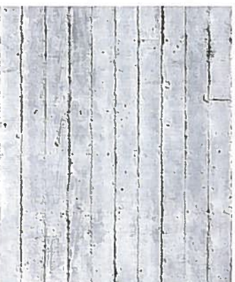
BOARD FORMED CONCRETE
