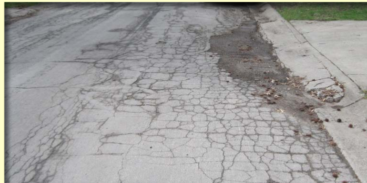
The Paving Program evaluates the 20+ miles of residential and collector streets in the Fair/Poor Category annually for mill/overlay improvements.
