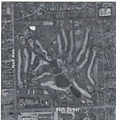
Aerial view of Meadowbrook Country Club property.
