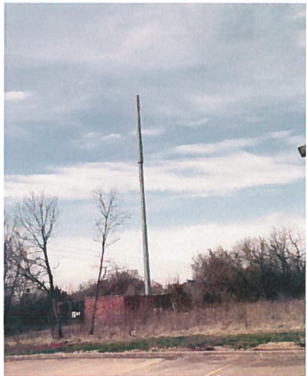
Existing Shrouded Antenna at 151 st St. & Switzer
