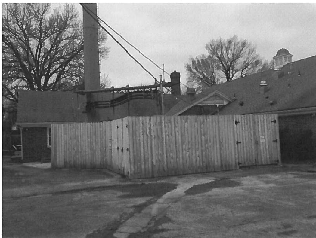
Equipment Compound (9011 Roe)
