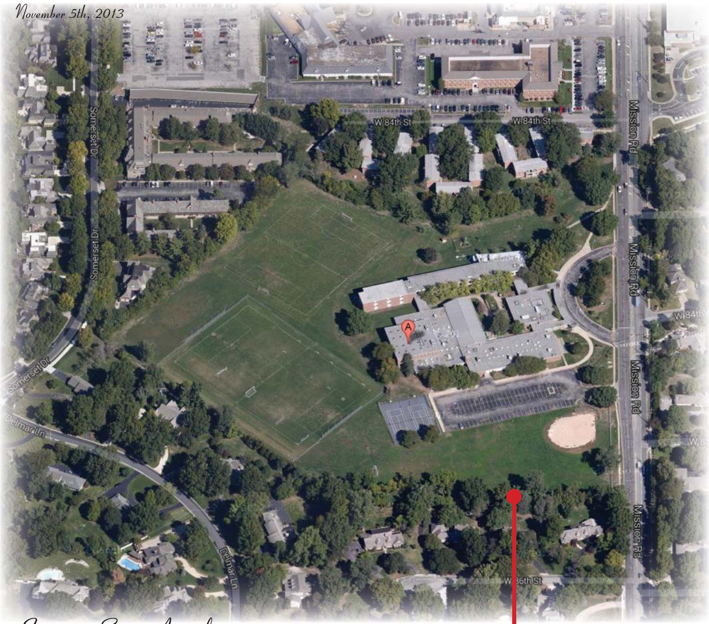
Existing Site Aerial
