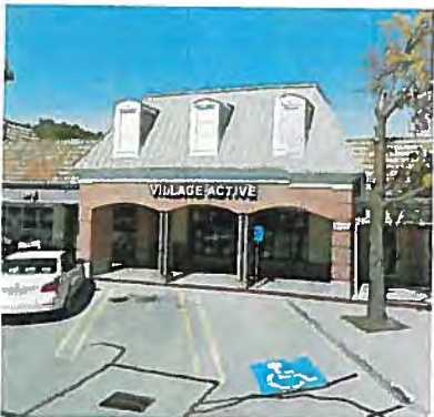
EXISTING EXTERIOR IMAGE E8
