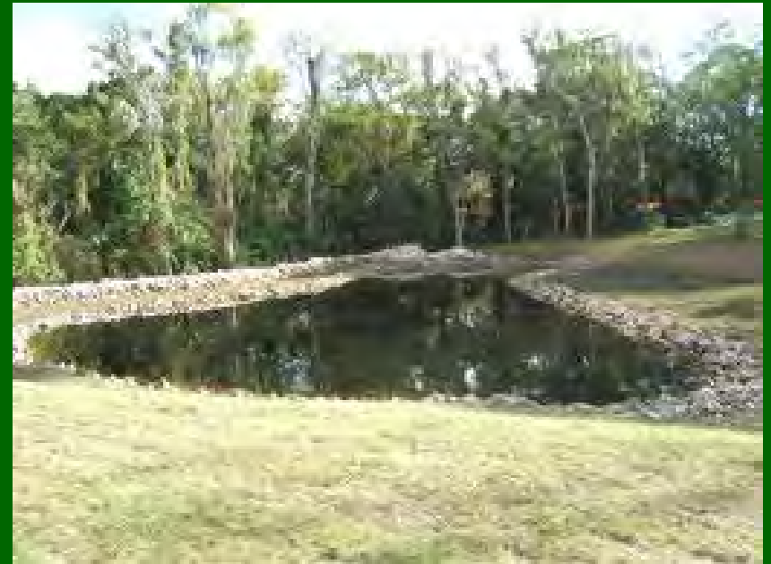
After Heavy Rain
