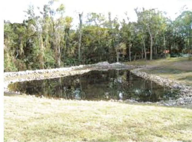
After Heavy Rain
