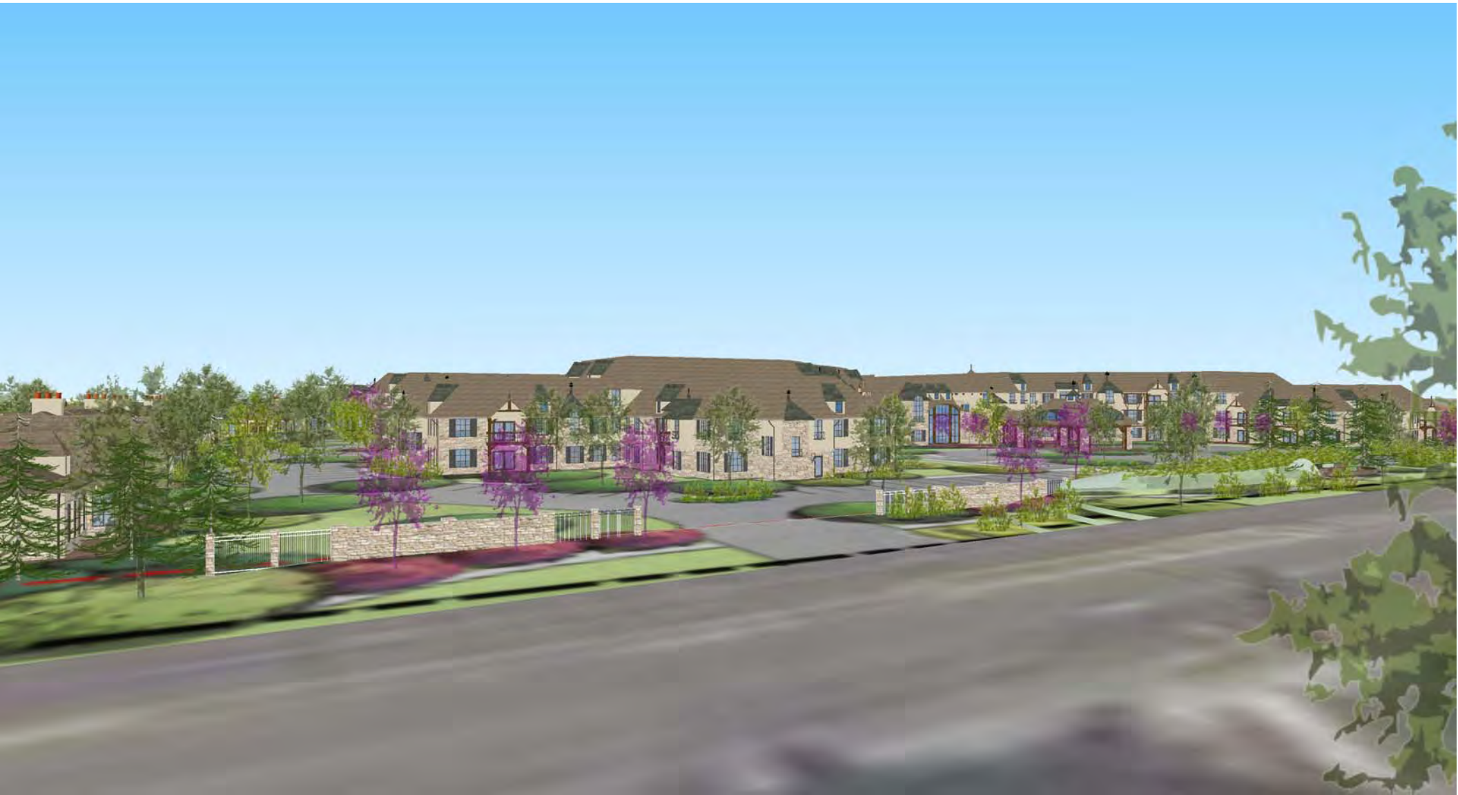
MISSION ROAD -LOOKING NORTHEAST
