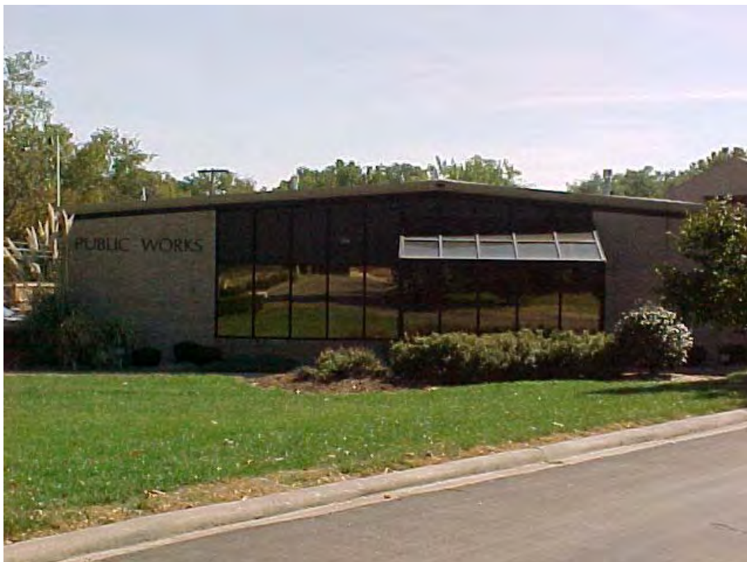
Public Works Office, 3535 Somerset Drive
