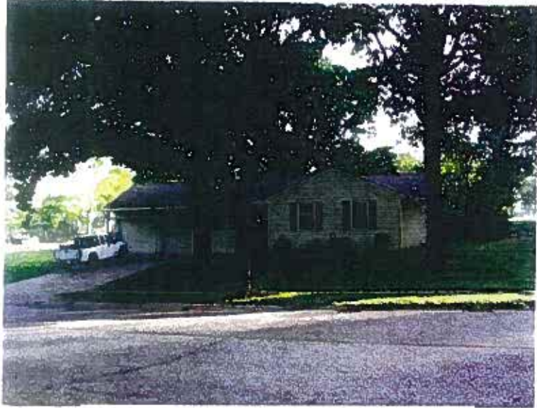
Adjacent Property to East
