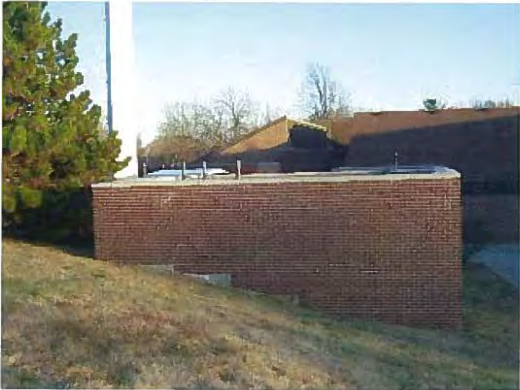
Equipment Compound (City Hall)
