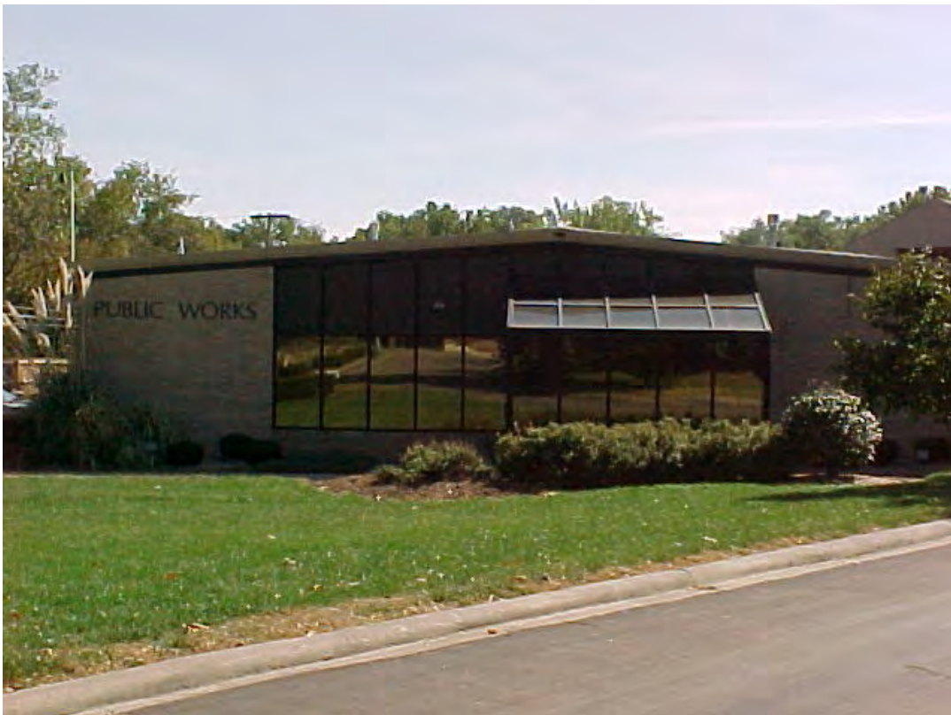
Public Works Office, 3535 Somerset Drive
