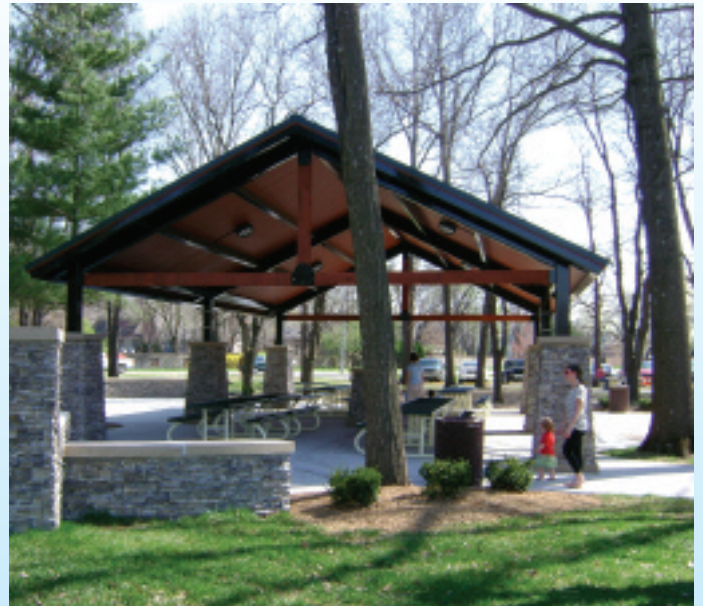
New Franklin Park Shelter (Somerset Ave. & Roe Ave.)
