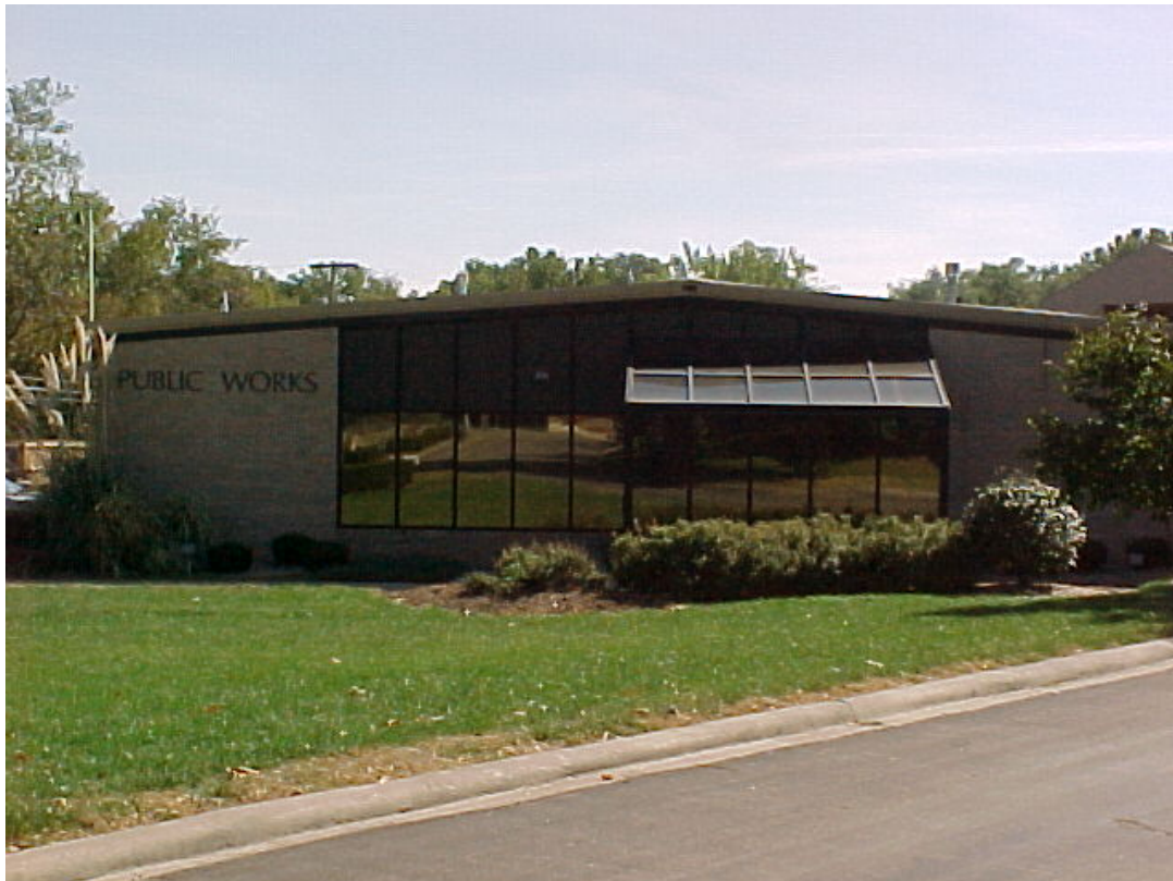
Public Works Office, 3535 Somerset Drive
