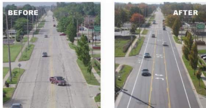
Figure 4: Road Diet - Before and After (Photo courtesy of Jennifer Selby)
