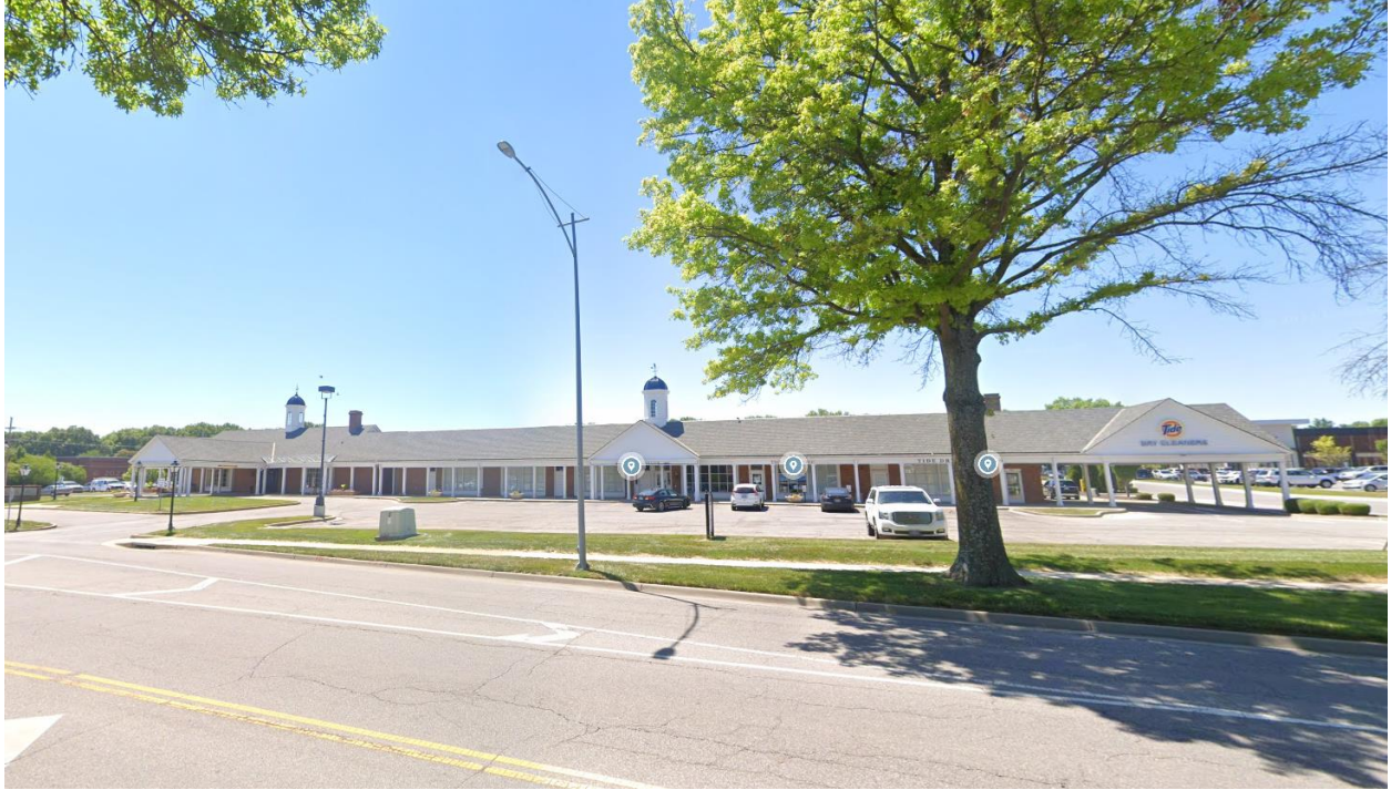
Looking southeast on 83 rd Street
