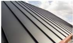
STANDING SEAM METAL ROOF
