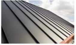
STANDING SEAM METAL ROOF
