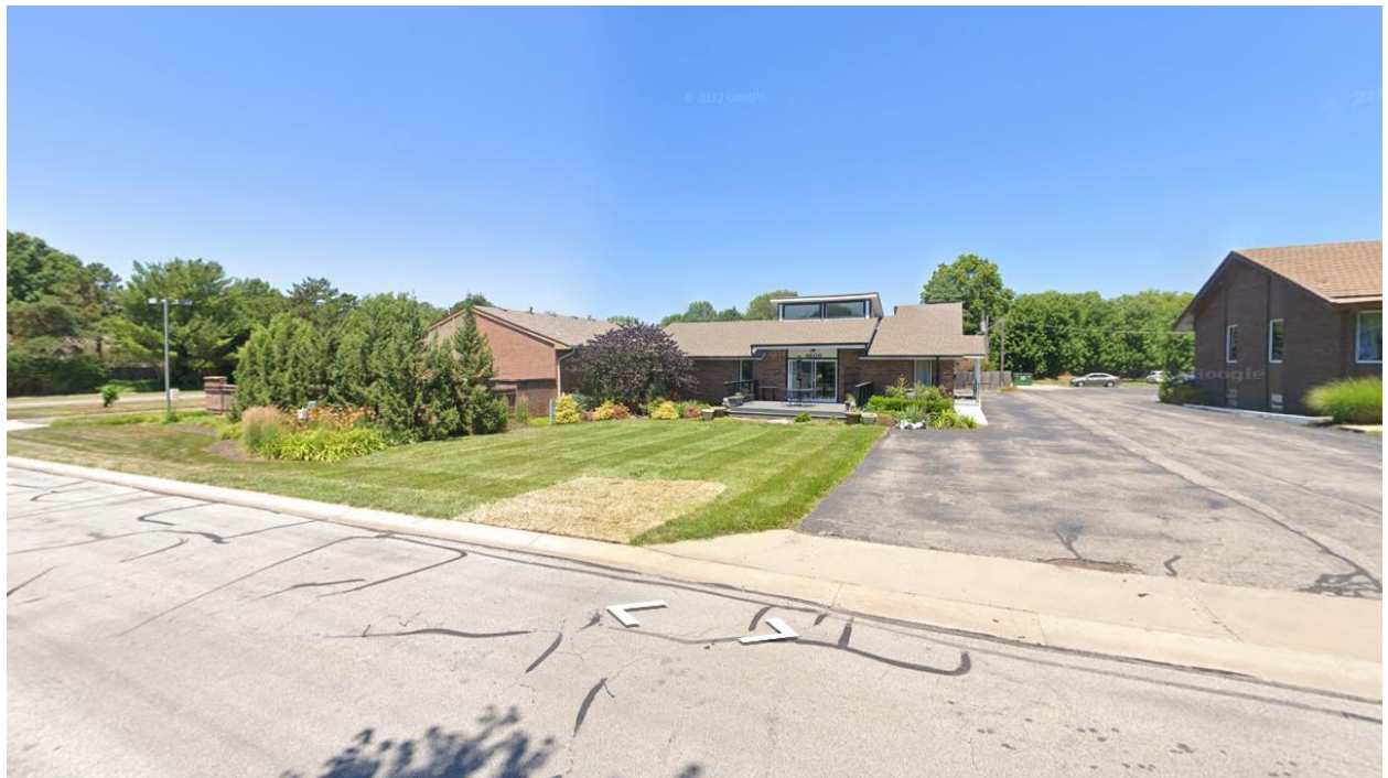
Street view looking north on W. 89 h Street
