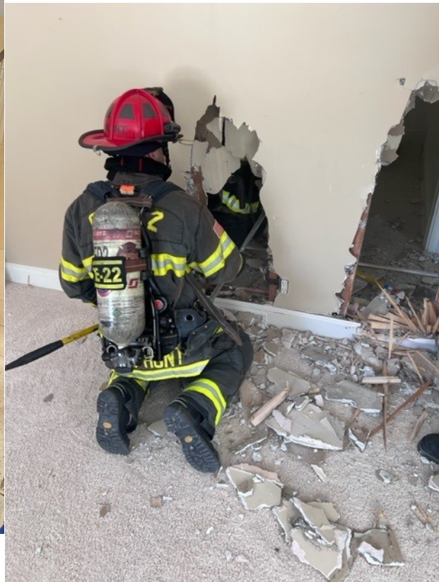
More fire operations training in the donated house. We are appreciative to the home owner for allowing CFD2 to train before they complete renovations. These donated homes allow CFD2 to train on actual tactics used in real life situations.
