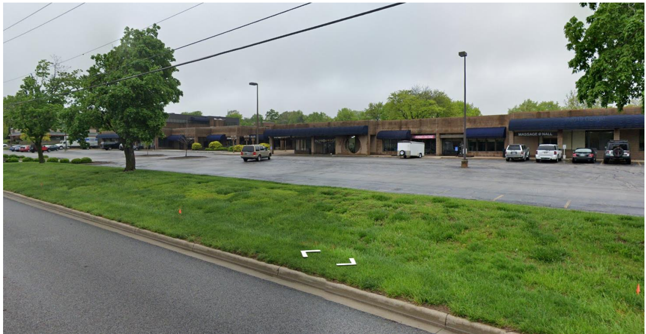
Street view looking northwest at the parking area and building frontage from W. 95 th Street
