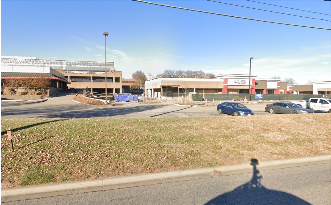
Street view looking north at from W. 95 th Street at the proposed ATM location prior to construction.
