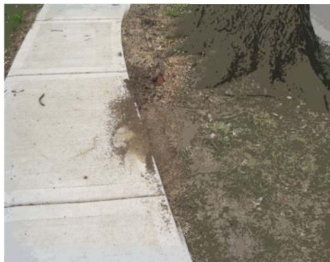
The Concrete Repair program focuses on a work area annually to repair curb/gutter and sidewalks.
