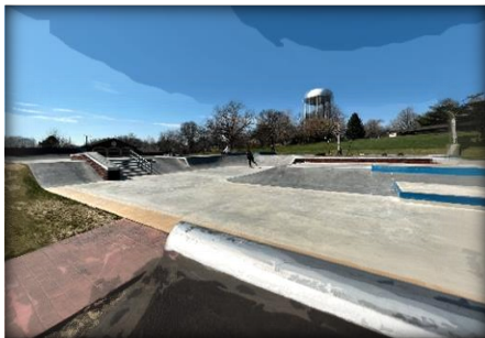
Lighting to be installed at these facilities.
