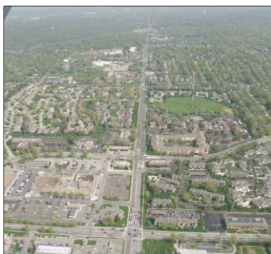
Aerial view looking north toward Corinth Square.
