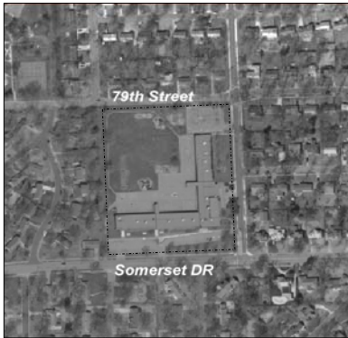
Aerial view of Somerset School site.
