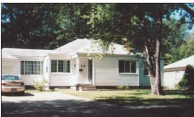
Typical ranch style homes with low - pitched roof and modest details.
