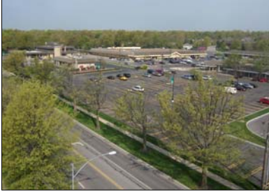
View looking west toward Corinth Square.
