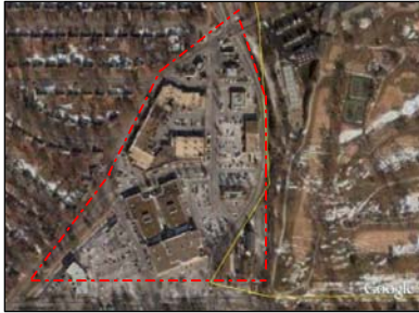
Aerial view of Prairie Village Shopping Center.
