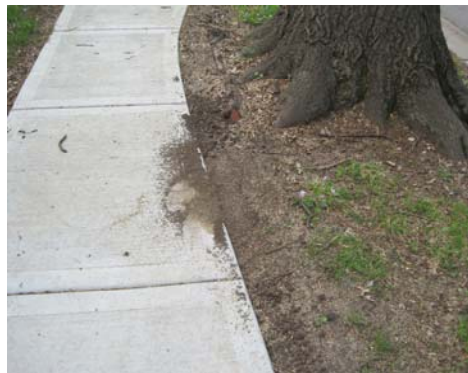
The Concrete Repair program sidewalk replacement focuses on a work area annually.
