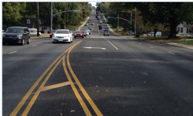
The UBAS program provides a maintenance solution for streets rated "good" between overlay treatments.
