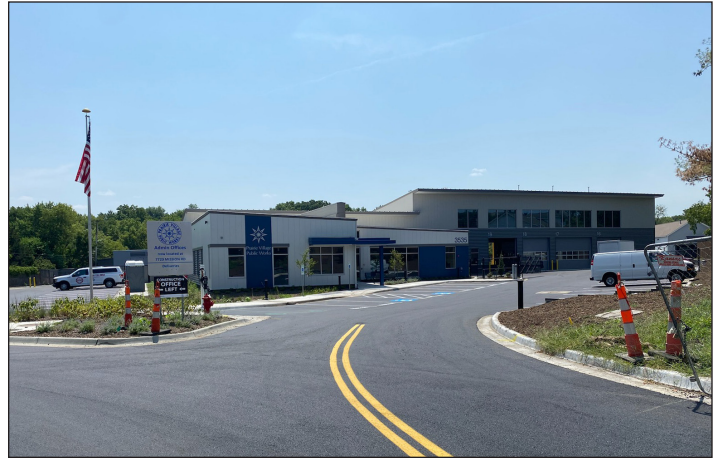
The newly-constructed public works facility
