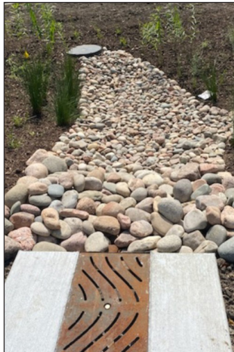
Rainwater collection system
