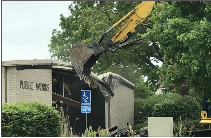
Prairie Village Public Works, 3535 Somerset during demolition
