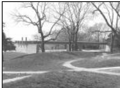
Harmon Park Pavilion
