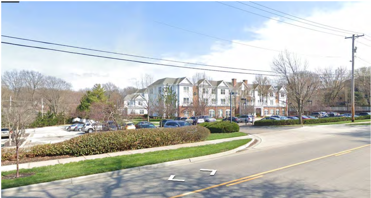
Street view looking east from Mission Road
