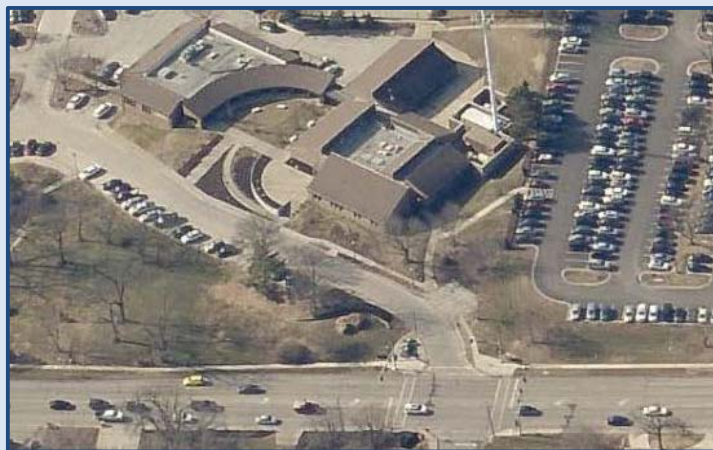
Replacing windows, doors and hallway carpet in City Hall.
