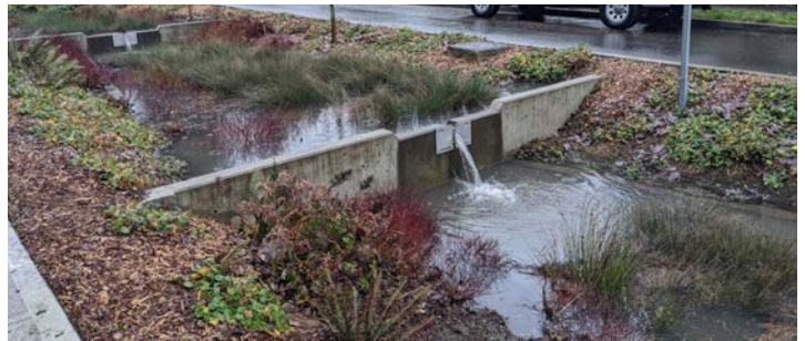
Bioswale | Broadview, WA
