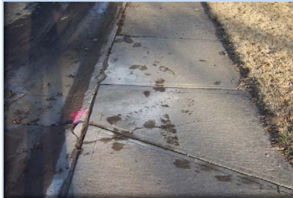
The Concrete Repair program sidewalk replacement focuses on a work area annually.
