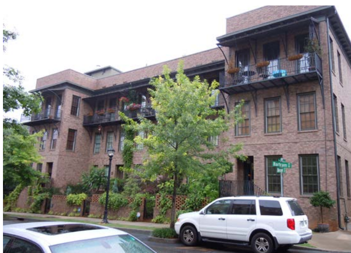
Small Apartment | Glenwood Park, GA
