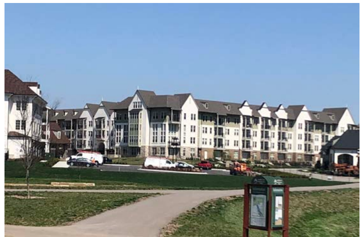
Apartment Building | Prairie Village, KS
