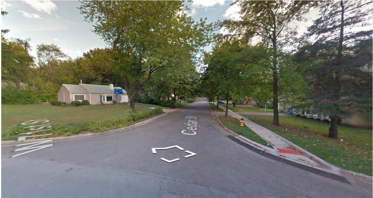
Street View (looking north on Cedar Street, subject property on left, prior to construction)
