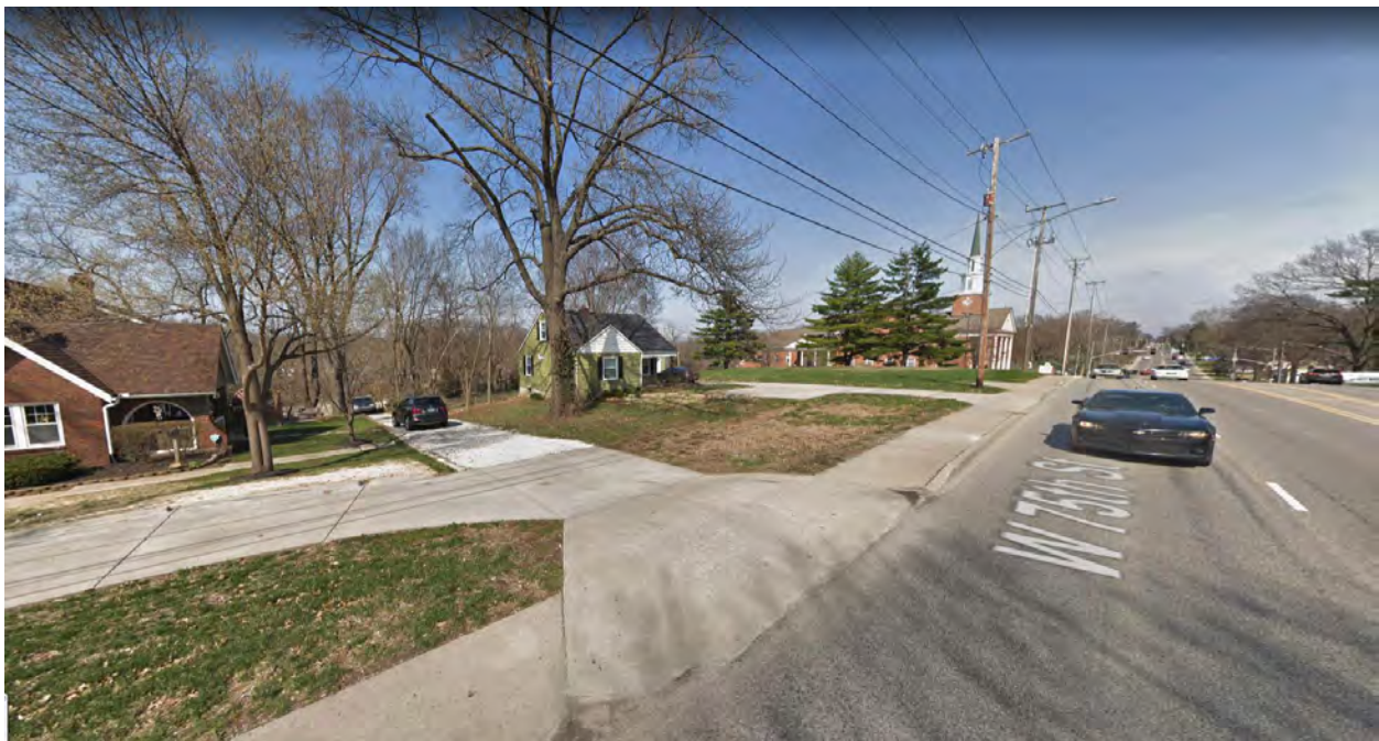
Street View (looking east on 75 th Street)
