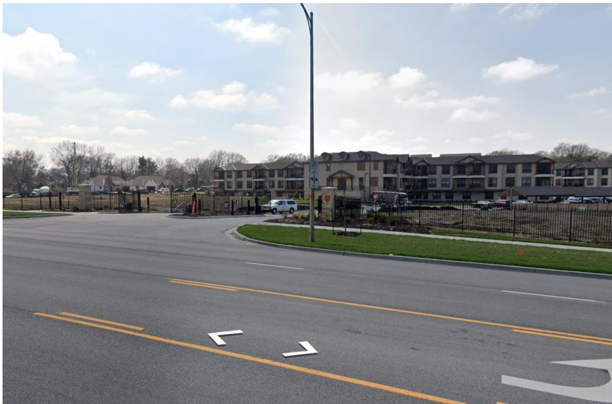
Street view at 8500 Mission Road looking southwest at entry.
