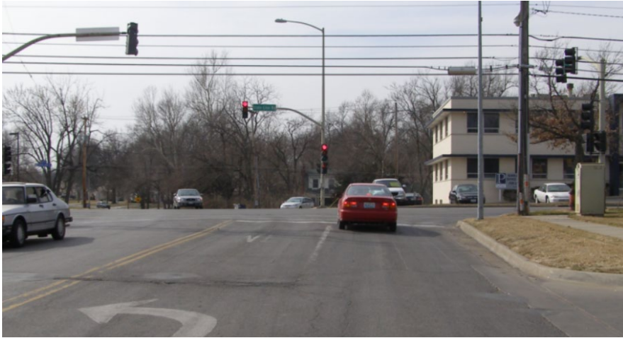
View looking west at the Somerset Drive and State Line Road intersection without signal backplates
