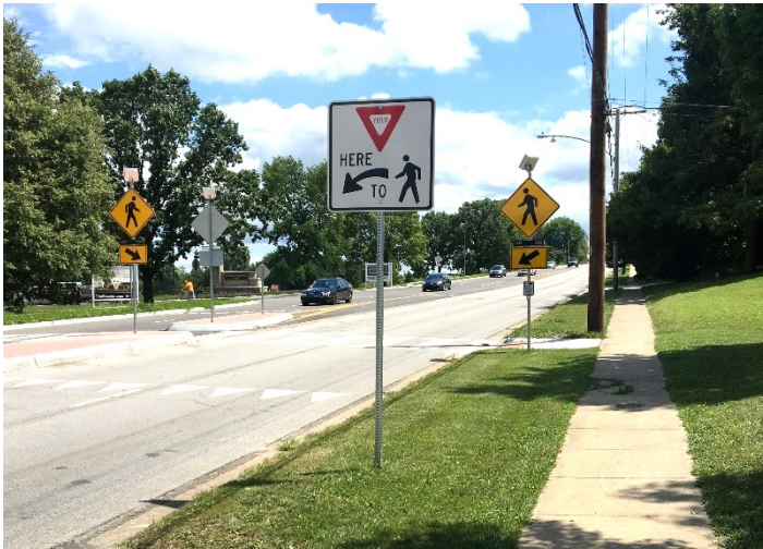
Rectangular Rapid Flashing Beacons (RRFB) installed on pedestrian crossing signage
