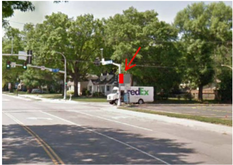
Red rectangle indicates location of recommended side-mounted signal head for southbound traffic at 71st Street and Mission Road
