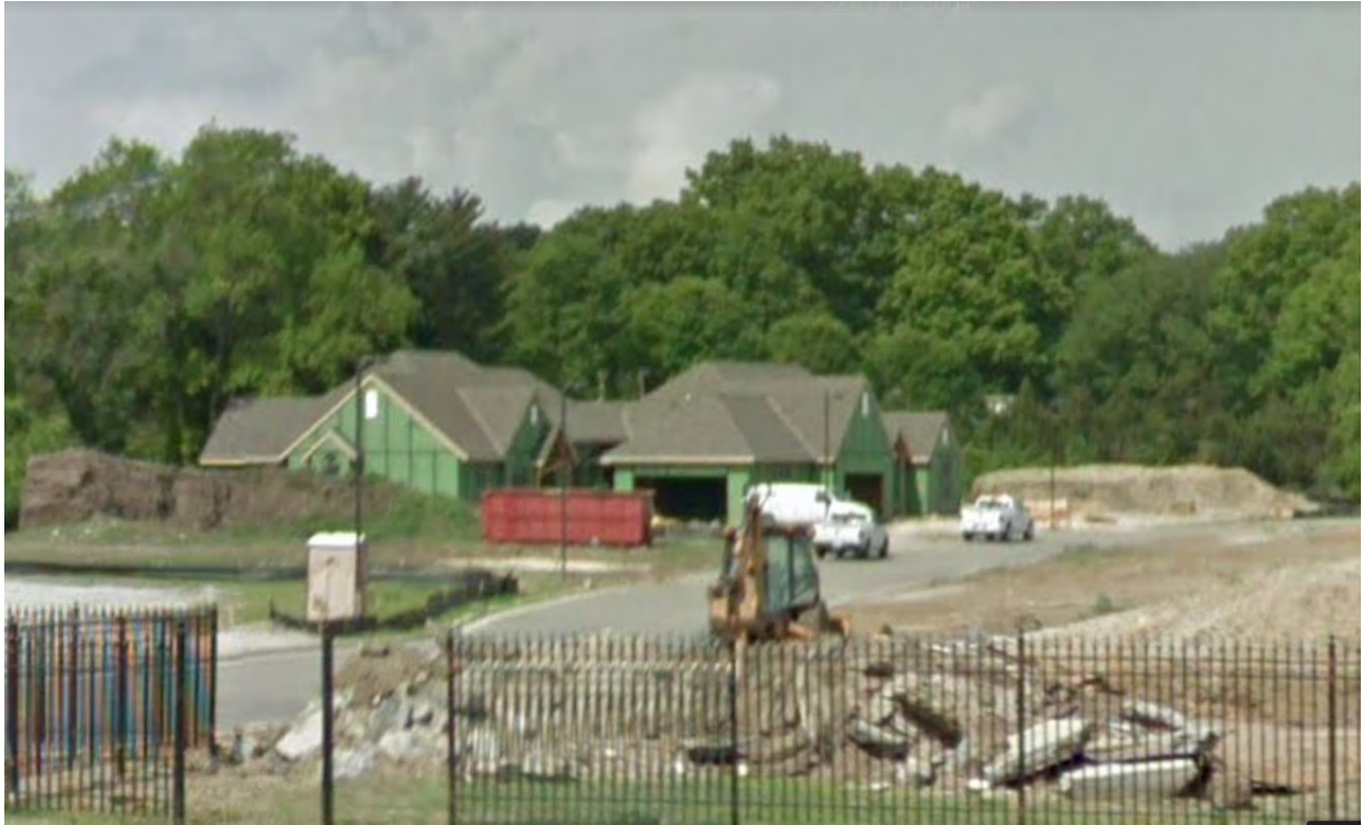
Street view looking west on Mission Road at 85 th Street
