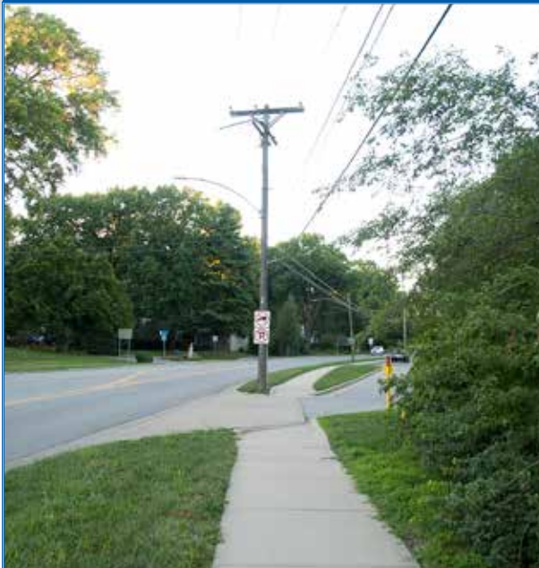
Figure 6. Mission Road utility poles and power lines
