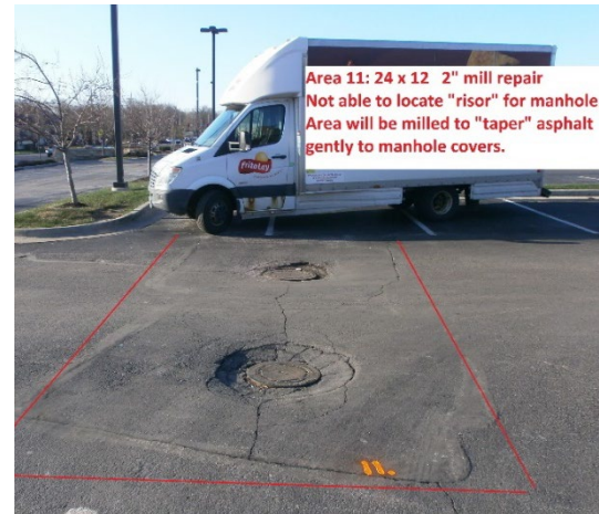
Parking lot repairs
