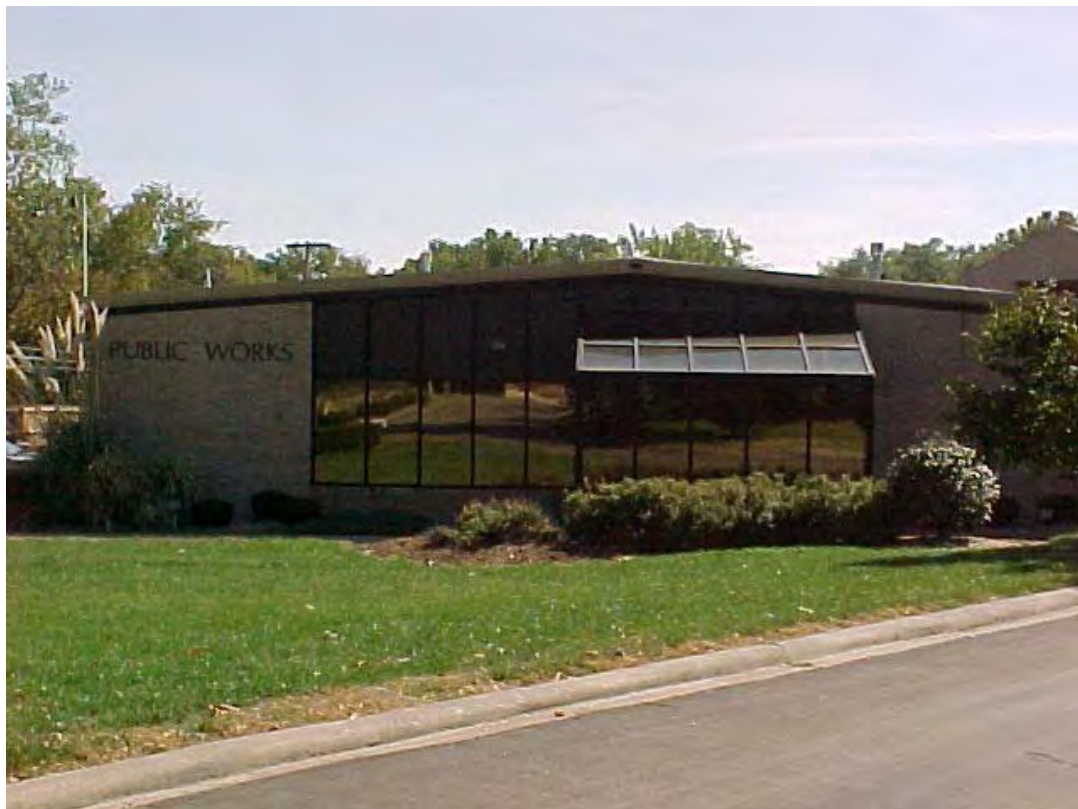
Public Works Office, 3535 Somerset Drive
